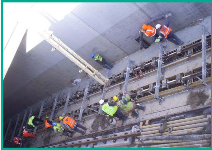
Track in Spine Road Underpass
