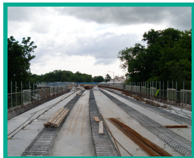
Brewery Road Bridge
