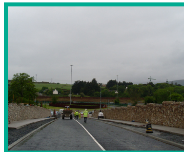
Glenamuck Road and Bridge works
