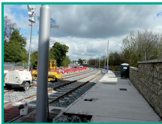
Installation of OCS - Blackthorne Avenue
